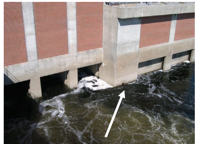
In Russian roulette, only one chamber has a bullet. At FPLE's Brunswick dam, downstream fish passage [small pipe at waterline] is sandwiched between multiple turbines. Just the opposite of the hand gun-gamble. Turbines here, of course, remain unscreened.
